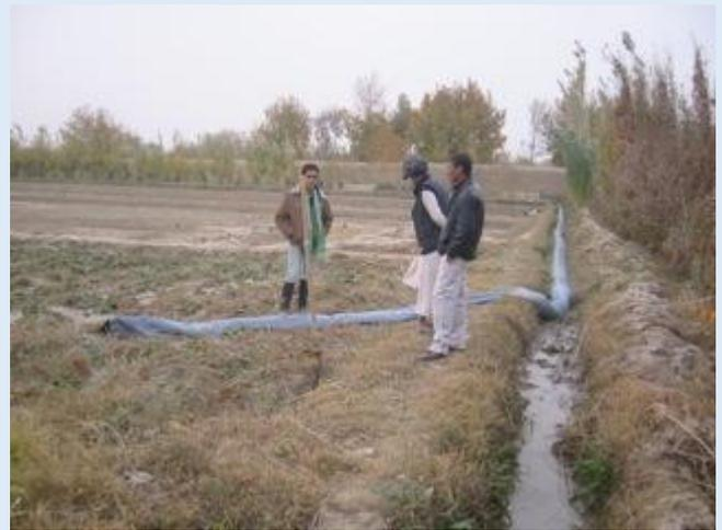
**Picture 8: Simple pipe turnout with siphon created from up-stream inline tarp intake**
