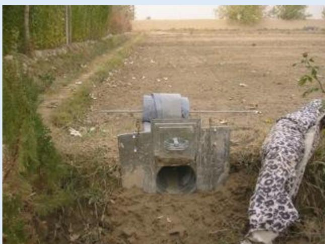
Picture 1: Inserting bank turnout with tarp
