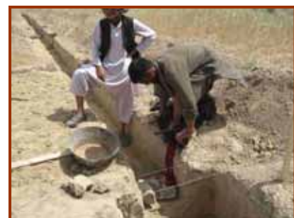
Making the sacrifice at the construction site.
